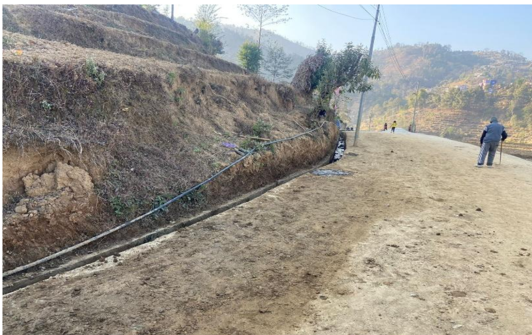
Debris Removal from Drain at Panauti Municipality-12, Badalpakha, Kavre
