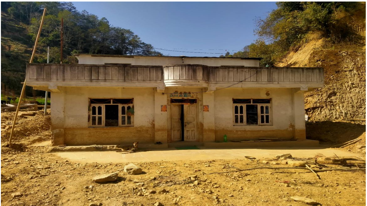
After - Debris Removal Works at Bethanchowk RM-4, Ganeshtan, Kavre
