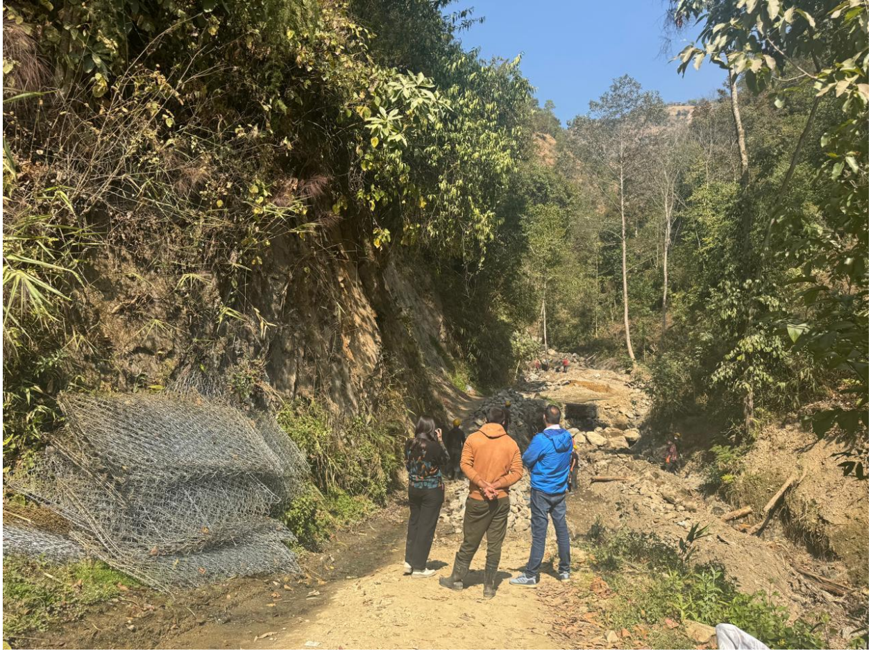
Gabion work in Mahankal
