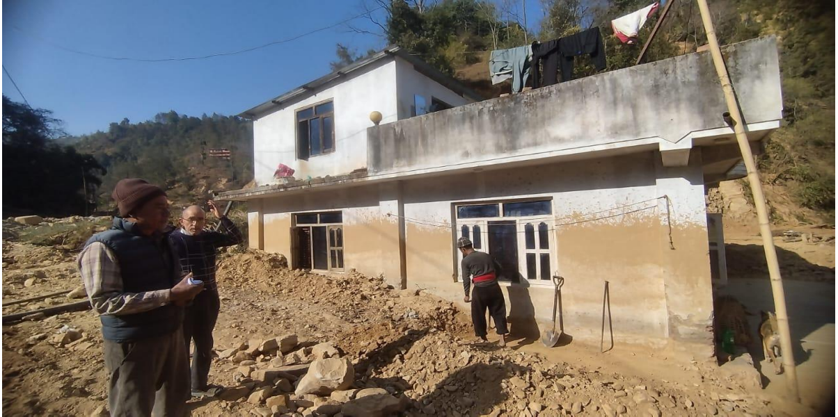
Debris Removal Works at Bethanchowk RM-4, Ganeshtan, Kavre
