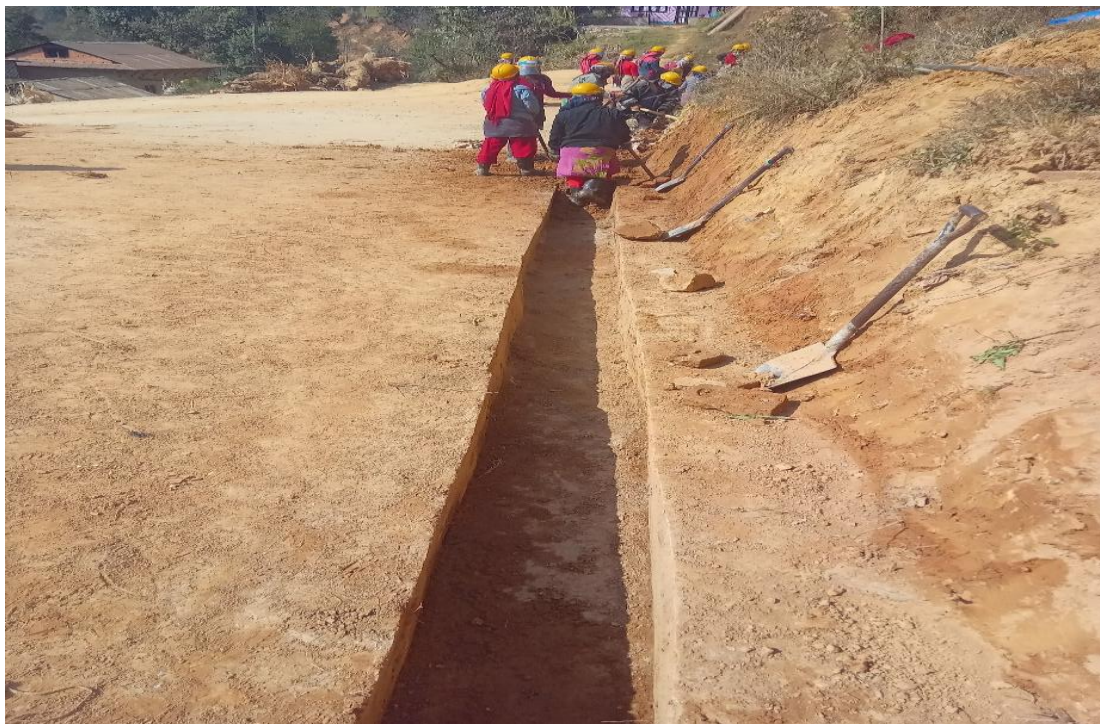
After Debris Removal of Drain of Panauti Municipality-12, Kavre
