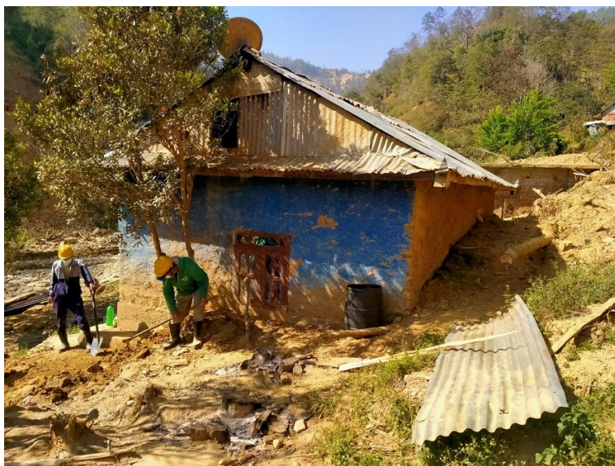
Before - Debris Removal Works at Bethanchowkl Rural Municipality-4, Pokharidada, Kavre
