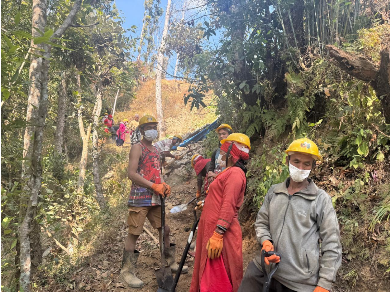
Work Progress in Mahankal
