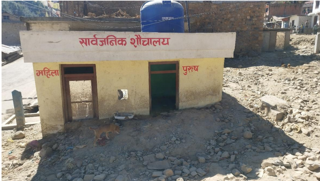
Before - Debris Removal Works at Bethanchowk RM-3, Dhungkharka, Kavre
