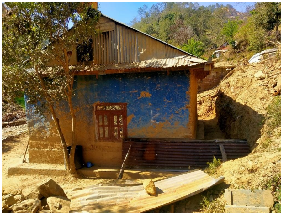
Debris Removal Works at Bethanchowk Rural Municipality-4, Pokharidada, Kavre
