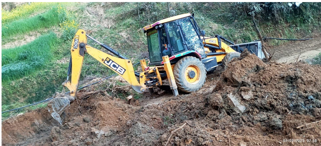
Removing the debris using an excavator
