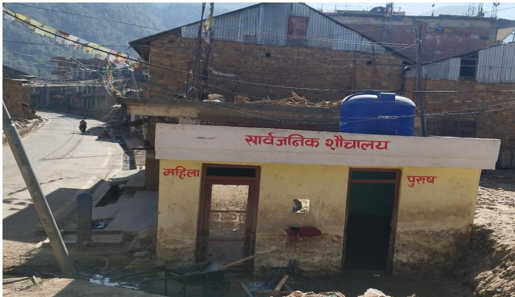
After - Debris Removal Works at Bethanchowk RM-3, Dhungkharka, Kavre
