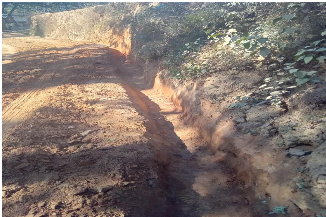
Debris Removal of Drain at Panauti Municipality-8, Ratopokhari, Kavre
